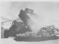
A ROCK contractor's dump truck is partly obscured by dust as it unloads into the rock crusher's hopper. DUMP TRUCK di un entrecador di piedra ta worde obscurci pa e stof ora e ta baha piedra den e garnador di piedra.
